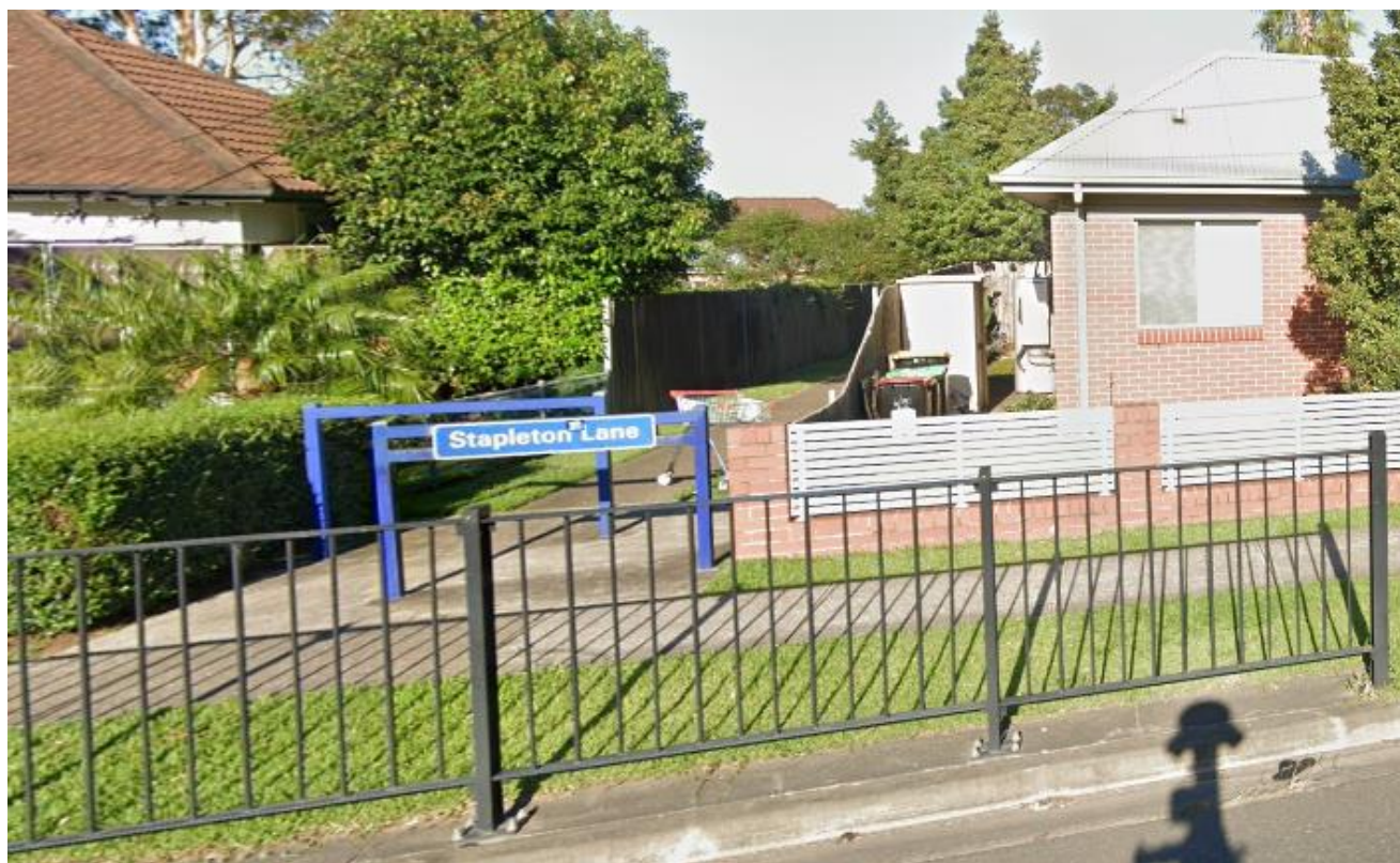
Barriers (in blue above) to be removed or adjusted for easier wheelchair access
